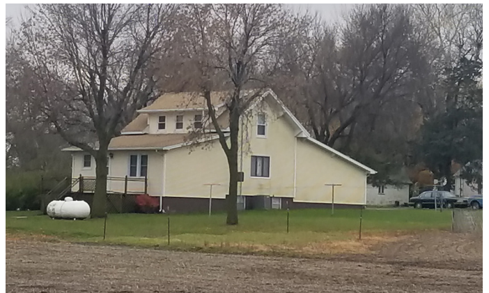
Figure 4.13: Yetter Housing Conditions
